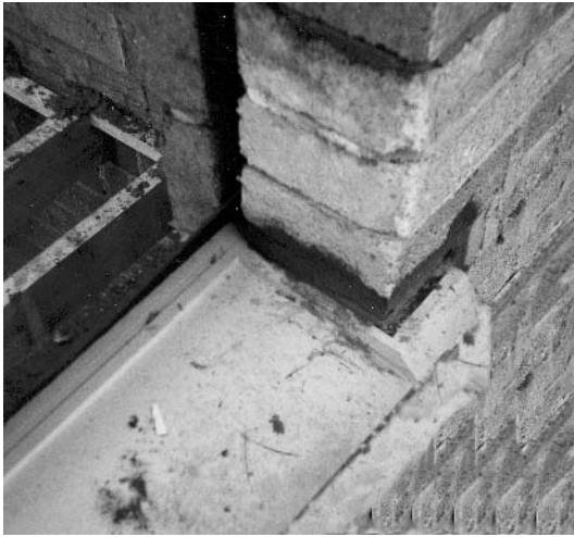
Fig. 5.7 Photograph of 1990s sill and jamb.
