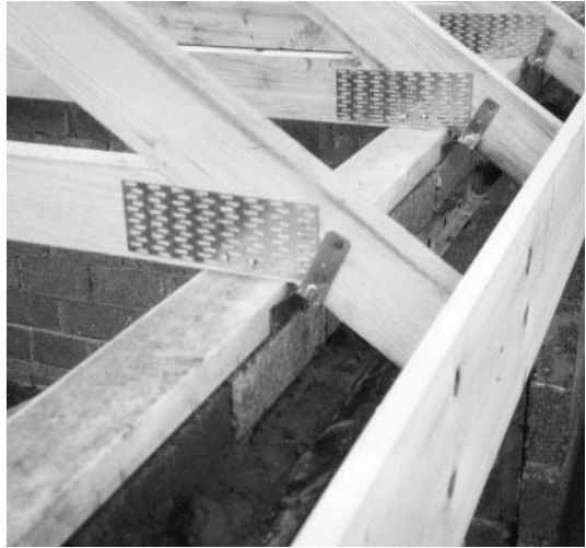
Fig. 6.16 Trussed rafters secured to wall plate.
