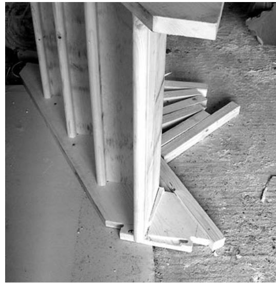
Fig. 10.8 Ends of stair stringers.
