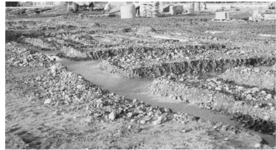
Fig. 2.1 Site with topsoil removed – concrete foundation in foreground.
