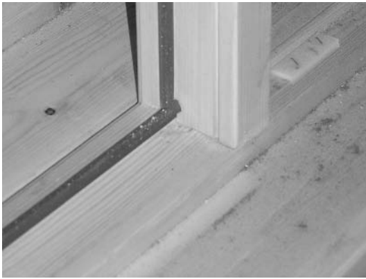
Fig. 9.13 Mullion and frame sill joint.
