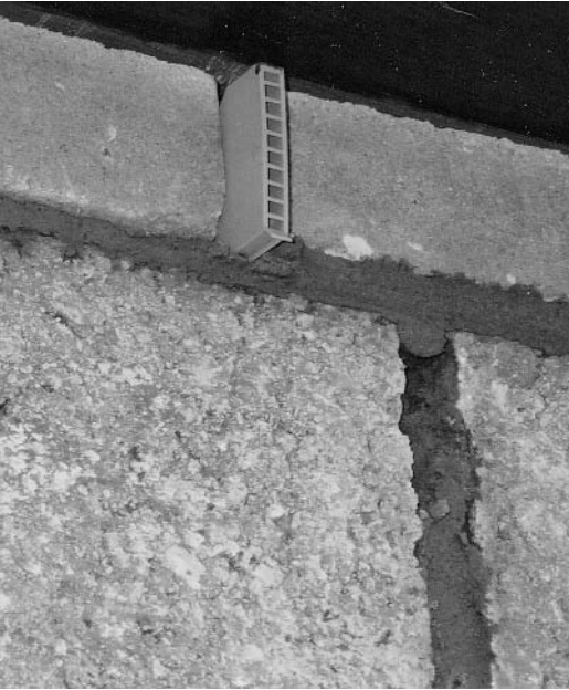
Fig. 3.21 Weep as a ventilator at the wallhead.
