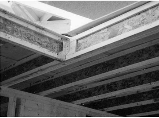
Fig. 4.32 Upper floor supported with Finnjoists.
