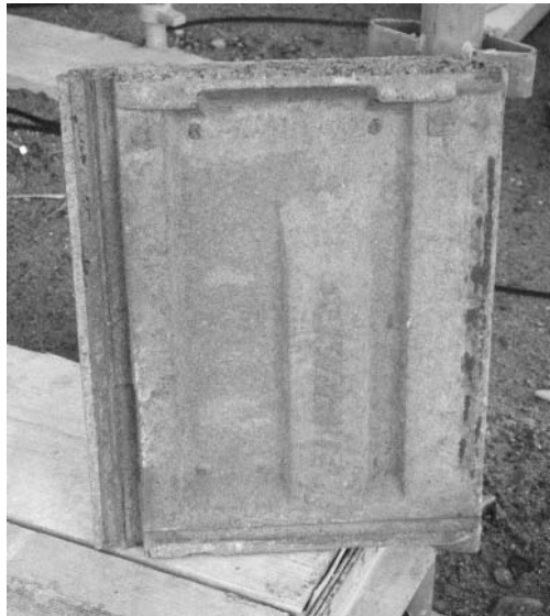
Fig. 7.6 Underside of an interlocking tile.
