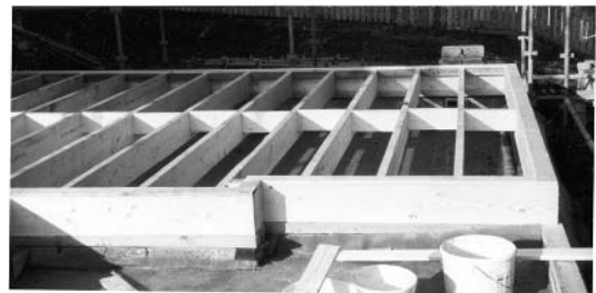
Fig. 3.25 A ring beam and joisted base ready for panel erection.
