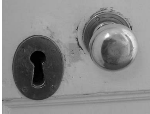
Fig. 8.19 The escutcheon plate for the lock in Figure 8.18.
