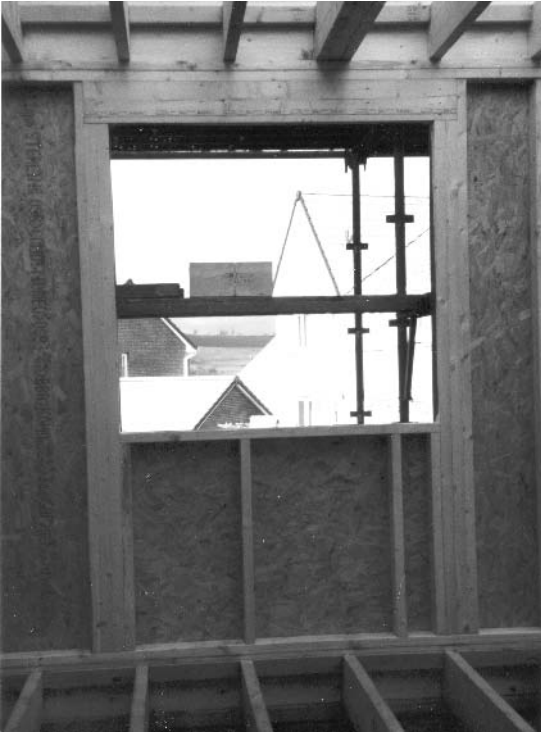
Fig. 5.41 Modern timber panel at window opening.
