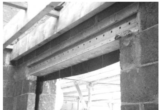
Fig. 5.10 Steel lintel at inner leaf of opening.
