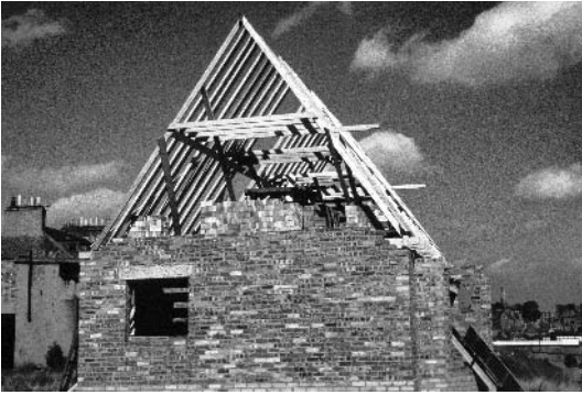
Fig. 6.34 Stick built roof (3).
