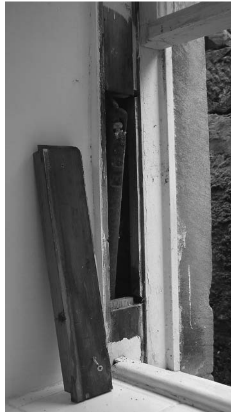
Fig. 9.27 Pocket in stile open.
