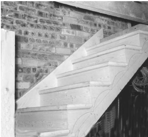
Fig. 10.3 Open cut string stair being installed.
