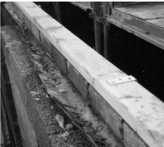
Fig. 6.15 Wall plate secured to wall head.
