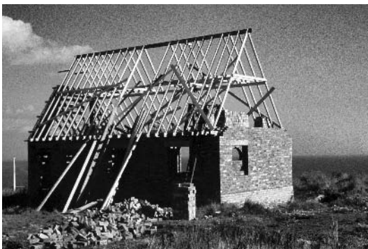
Fig. 6.31 Stick built roof (1).
