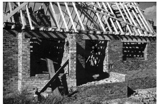
Fig. 6.33 Stick built roof (2).
