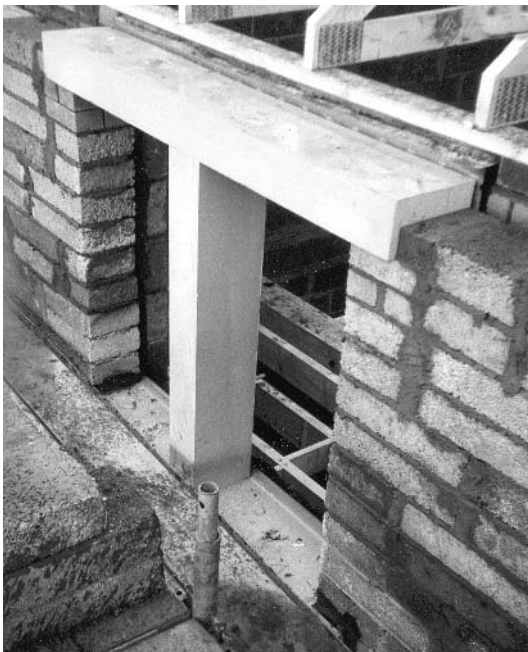
Fig. 5.8 Photograph of 1990s head, sill and mullion in artificial stone.
