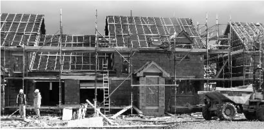
Fig. 7.1 Houses ready for roof tiles.
