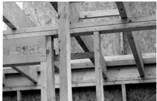
Fig. 4.7 Upper floor joists supported by a partition (2).
