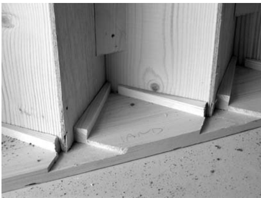
Fig. 10.7 Step to stringer joint.
