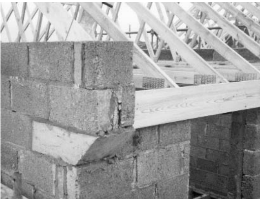
Fig. 6.35 Corbel at eaves verge junction.
