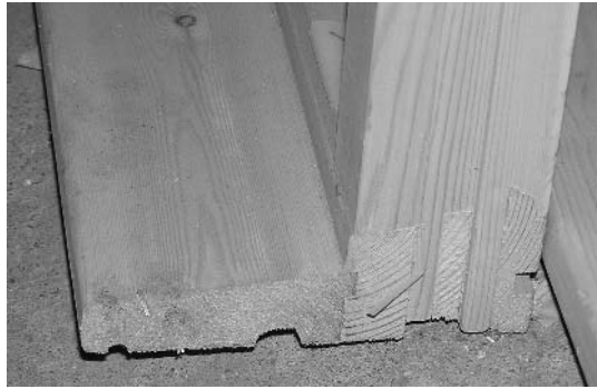
Fig. 9.11 Casement sill and frame stile joint.
