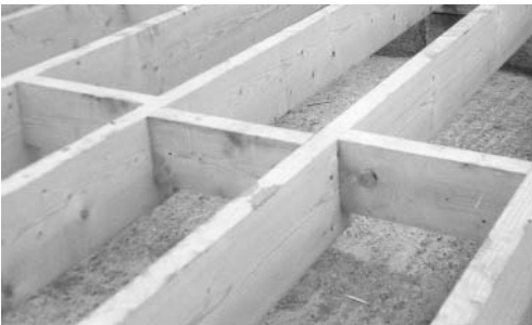
Fig. 4.17 Solid timber strutting.
