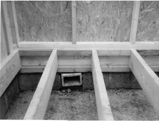
Fig. 3.26 Panels erected on a base.
