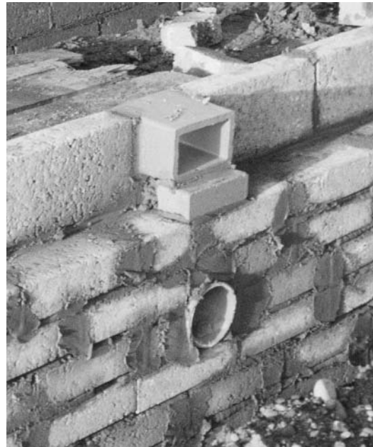
Fig. I.12 Terracotta liner built into a blockwork substructure wall.
