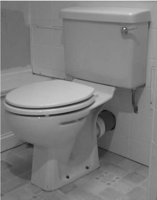
Fig. 12.39 Close coupled flushing cistern and WC.
