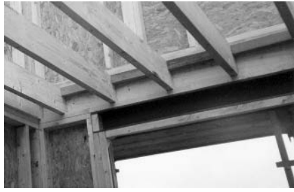
Fig. 4.5 Upper floor joists in timber frame construction (2).
