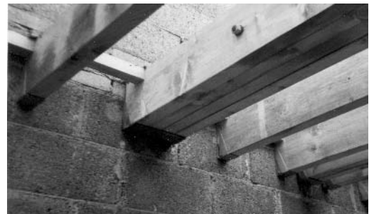
Fig. 4.3 Heavy gauge joist hangers supporting upper floor joists.
