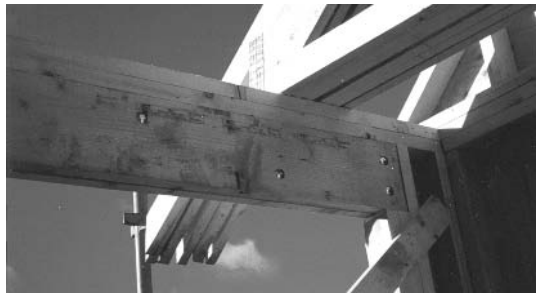
Fig. 5.44 Flitched beam over large opening.
