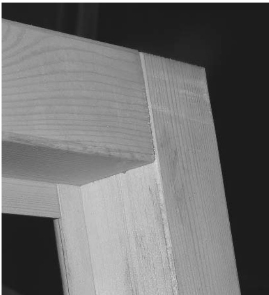
Fig. 9.14 Casement joint.
