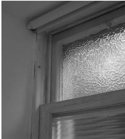
Fig. 9.24 General view of sash and case window.
