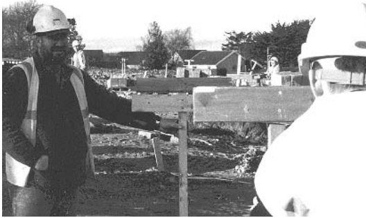
Fig. 2.35 Banksmen and traveller between profile boards.
