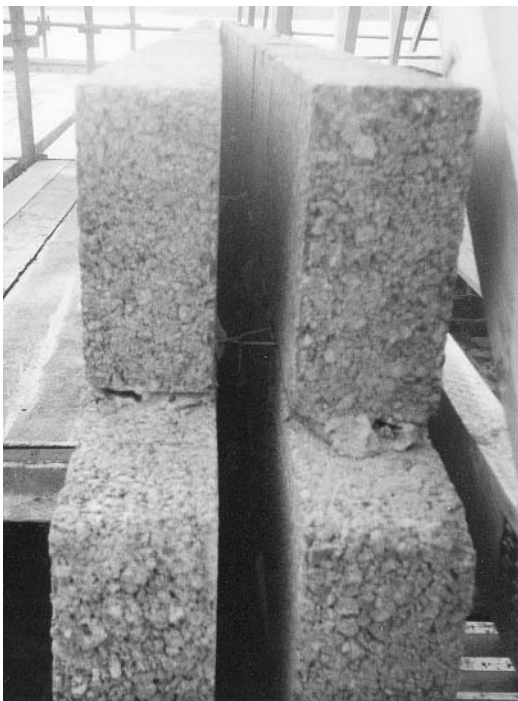
Fig. 3.5 Block cavity wall.
