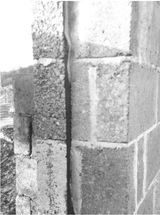
Fig. 5.11 Detail of checked jamb.
