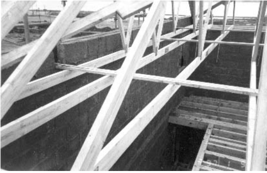
Fig. 6.14 Trussed rafter roof.
