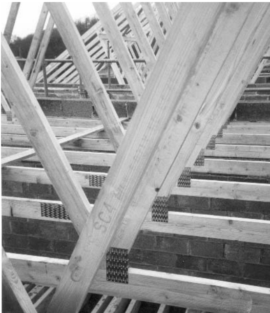
Fig. 6.17 View down centre of trussed rafters.
