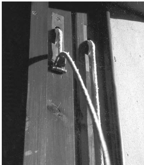
Fig. 9.25 Sash pulleys and cord grip.
