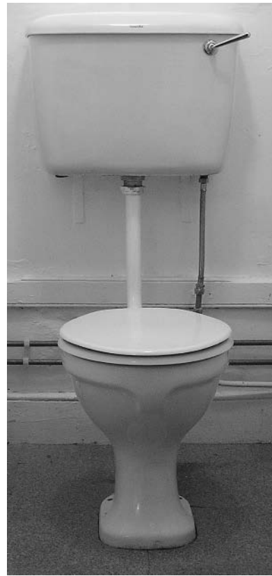
Fig. 12.38 Low level flushing cistern and WC.
