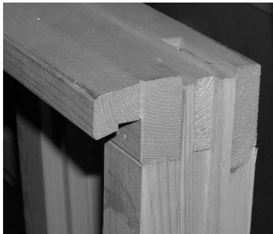
Fig. 9.12 Casement head and frame stile joint.
