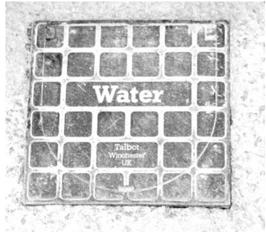
Fig. 12.25 Cast iron toby cover in the street.
