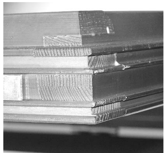
Fig. 9.9 Finger joints in a casement.
